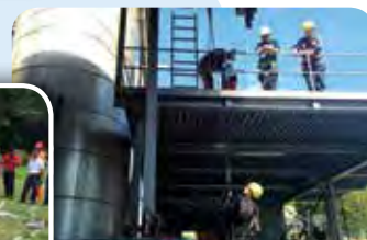
Workplace safety training such as working at heights was conducted at Kolb for all engineers
